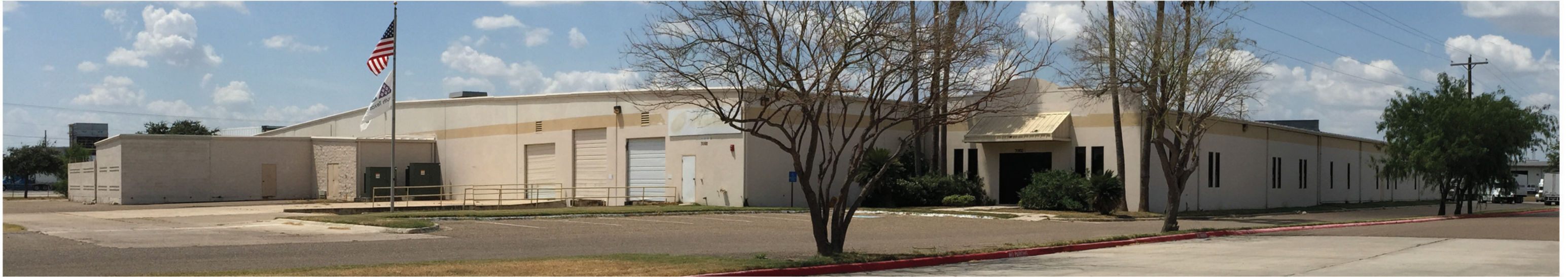
SOUTHEAST VIEW (VIEW FROM MILITARY HIGHWAY)
