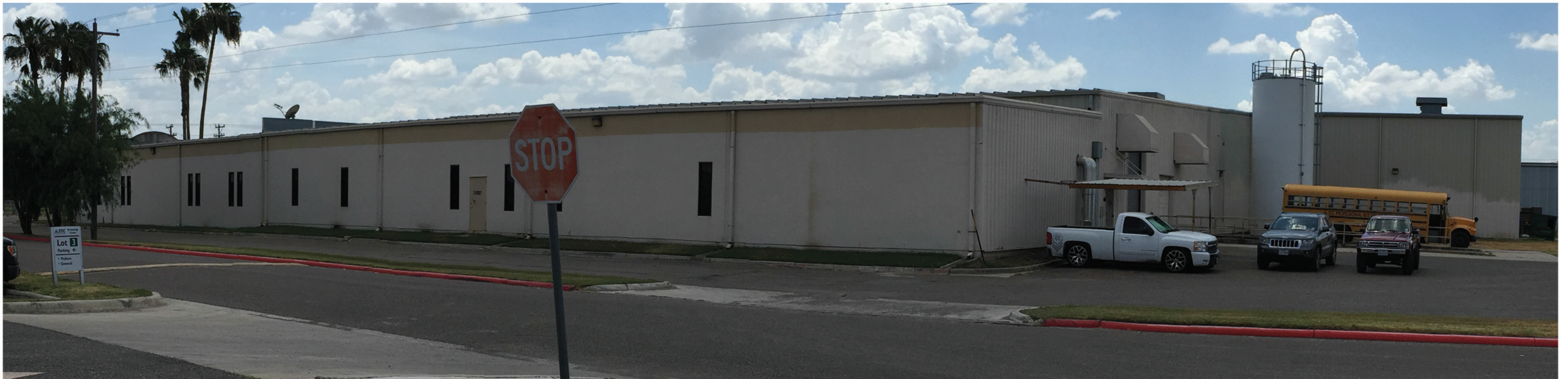
NORTHEAST VIEW (VIEW FROM BASKETBALL COURT)
